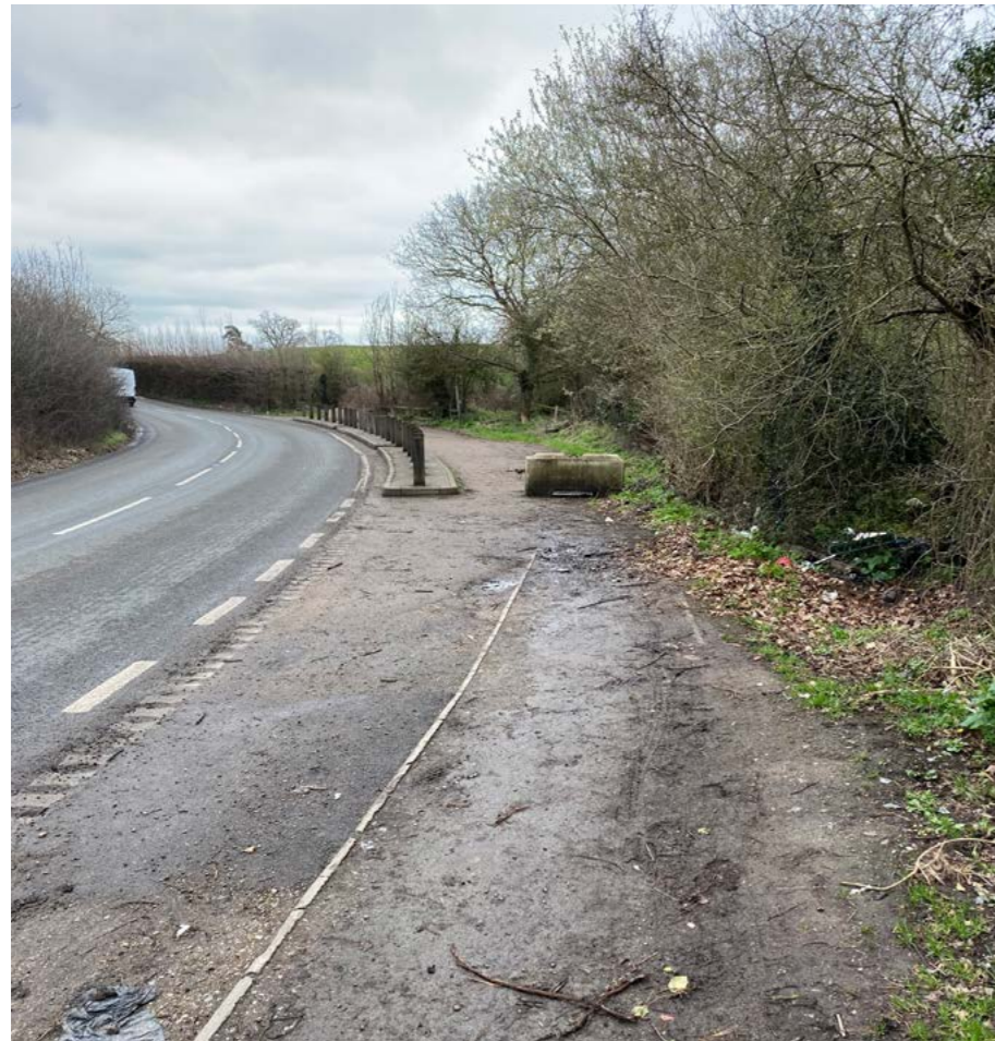
A FIGURE 130. View of Existing Lay-by
