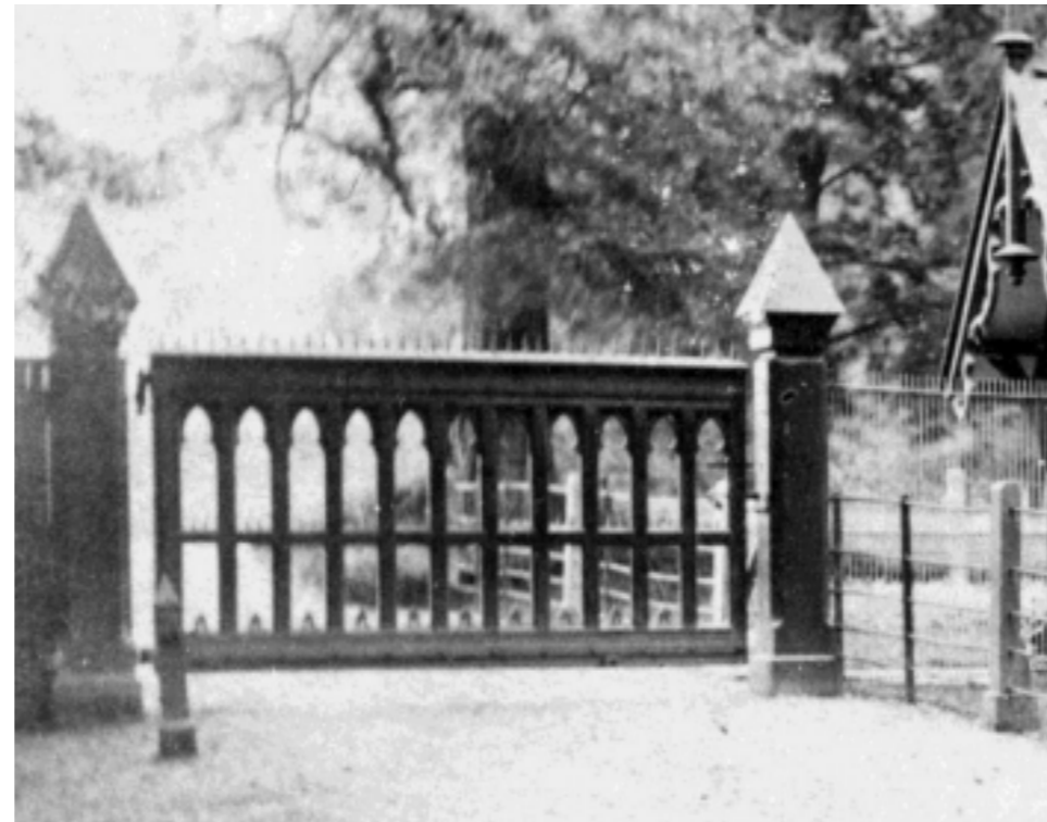
FIGURE 140. Historic Image of South Lodge Gate
