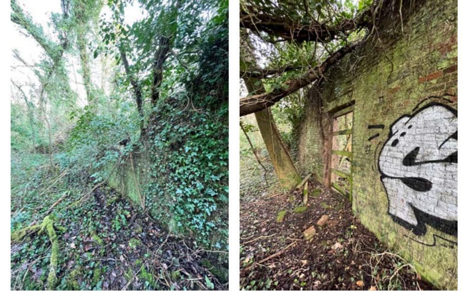
FIGURE 12. Existing condition of Historic Garden Wall
